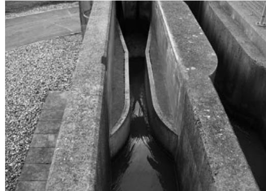
Venturi flume: Typical 3/2 power law
